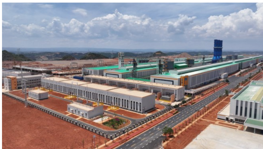
Figure 11. NEUI600 potlines under construction in Yunnan Honghe aluminium smelter.
